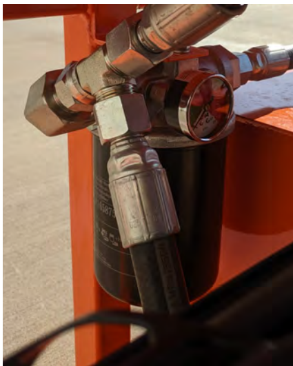
Figure 7: Hydraulic Fluid Filter
