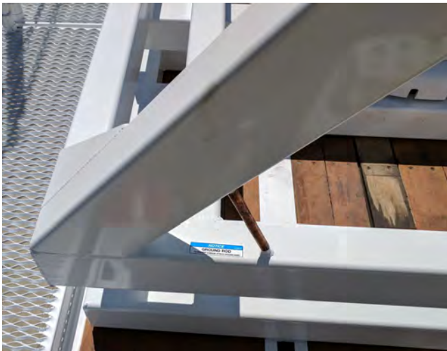
Figure 8: Ground Rod Locations
