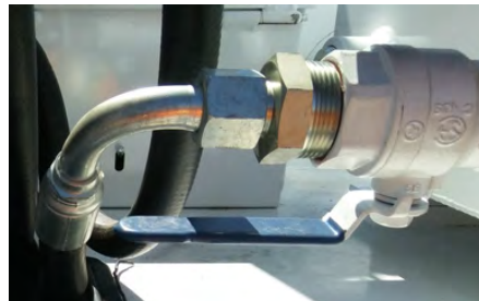
Figure 6: Oil Reservoir Shut-off Valve
